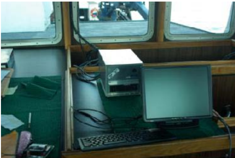
Figure A1. EM control box and user interface installation.
